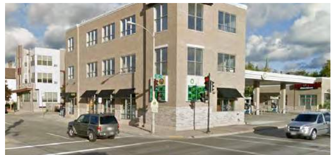
Figure 660(7) Fueling Pump Location
