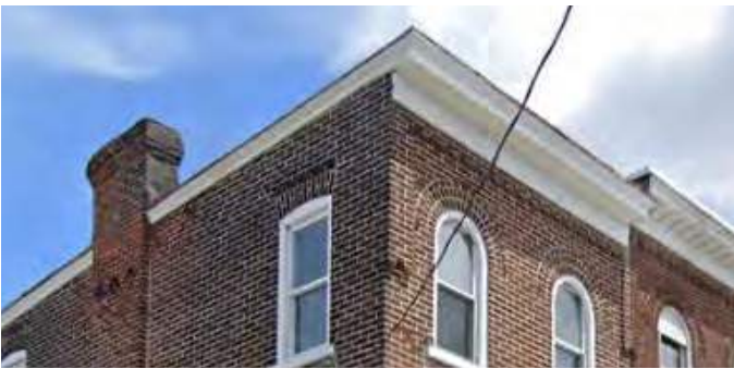
Flat Roof Type (with Cornice)
