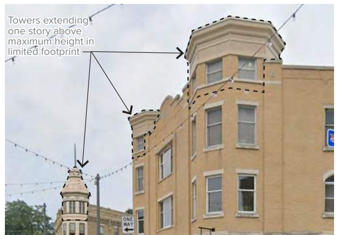
Figure 660(12) Example Towers Extending above Roofline
