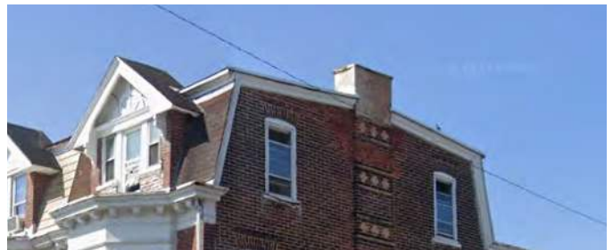
Pitched Roof Type (Gambrel Roof)
