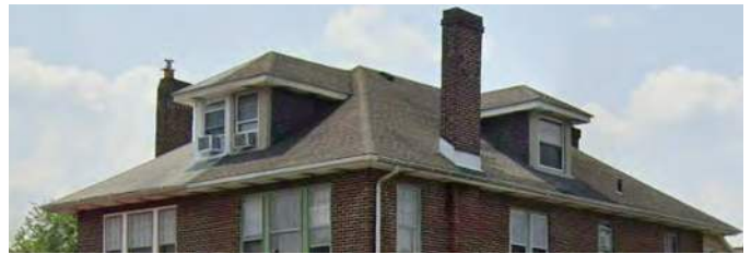
Pitched Roof Type (Hipped Roof)
